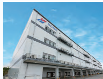
Kansai II Medical DC (Operation started in February 2018)
