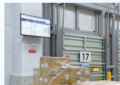
Monitor placed in loading dock
