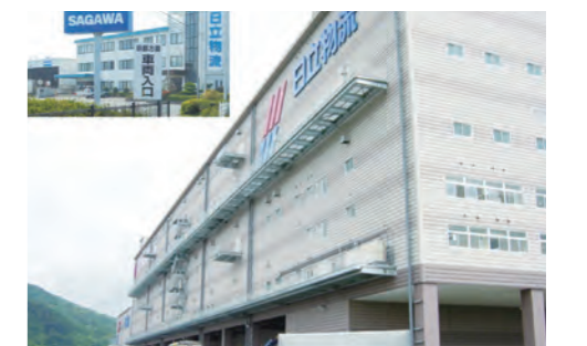
HTS Group Oyamazaki AE sales office (top left: sales office of SAGAWA EXPRESS)
