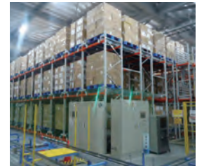
③ High-density storage system
