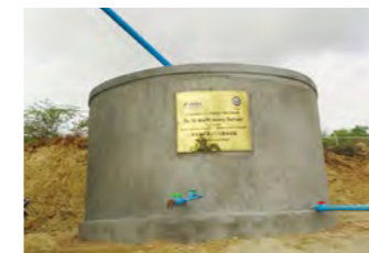
Example of support activities Supported "Children's Forest" Program of the Organization for Industrial, Spiritual and Cultural Advancement (OISCA) (public interest incorporated foundation), to install rainwater harvesting systems (Za Ya Ma Primary School/Myanmar)
