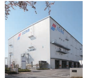
"R&D Center" (Fourth floor in existing distribution center)
