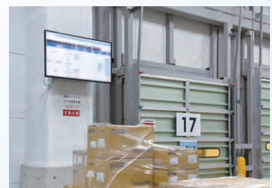
Monitor placed in loading dock
