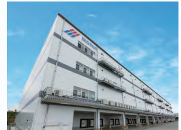
Kansai II Medical DC (Operation started in February 2018)
