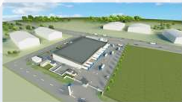
Nilai Cold Warehouse/Malaysia (Operations to be started in Nov. 2018)
