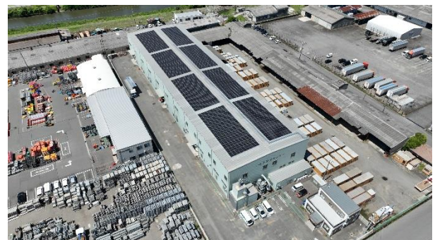
Power generation facilities at our warehouse
