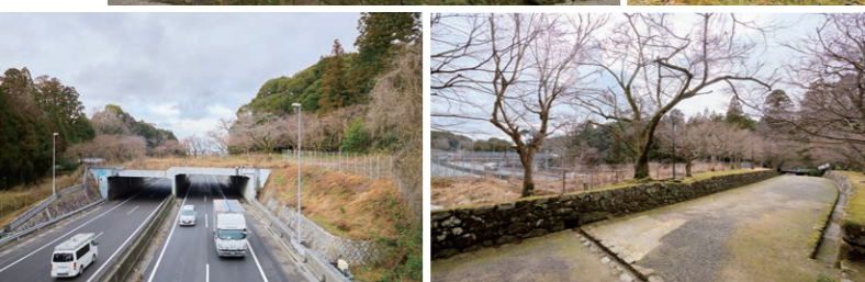
This area is near the approach to Saimyo-ji Temple, which is one of the three temples located around Lake Biwa, at Shiga Prefecture. The Main Hall and the three-storied pagoda have been named national treasures. Note the Meishin Expressway (bottom left photo) under the temple approach (bottom right photo). The Japan Road Group (as it was known at the time) designed the road so as to maintain this view.
