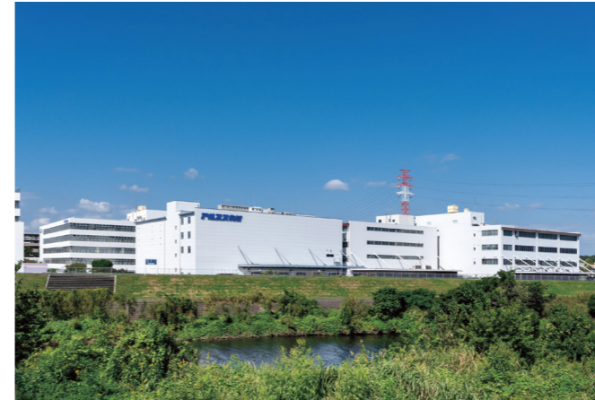
ALPS LOGISTICS Headquarters, located in a natural environment in the suburbs of Yokohama
