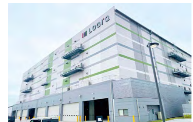
Kumiya Sales Office of Hitachi Transport System West Japan Co., Ltd.
