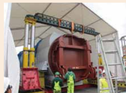
Installing transport connector attachments
